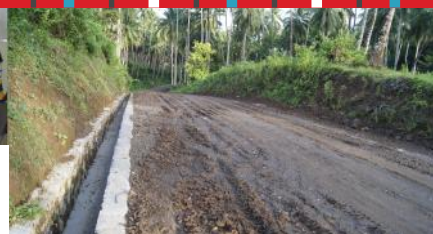
Tubod, Surigao del Norte - Rehabilitation of Farm-to-Market Road (Graveling of Road with Concrete Canal)
